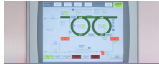
Control Panel/ PLC/ VFD Retrofits
